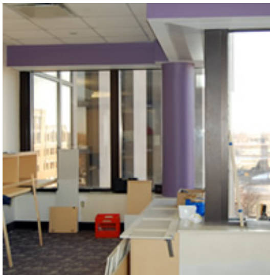
MetroHealth Family Room under construction.
